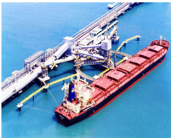
Figure 2. Material handling system including marine structures and shiploaders designed to handle either molten or prilled sulfur.
