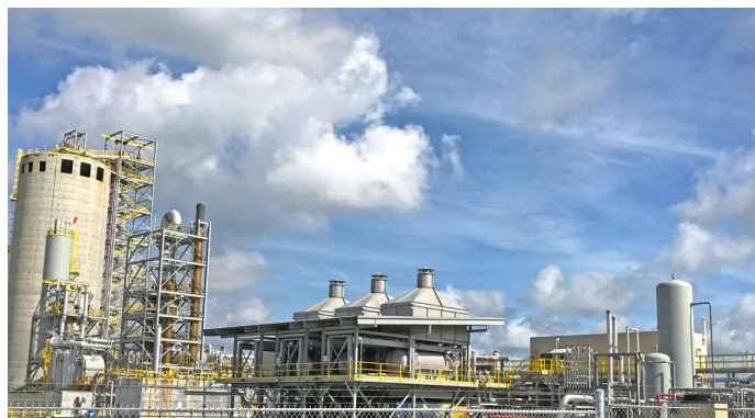
Figure 4. Three modular pressure leaf filter units at a 1 million tpy sulfur remelting facility.
