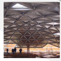
to your specifications, including design loads, to provide maximum protection and asset life with minimum maintenance expense. The dome and any modules such as platforms, bird screens, skylights or inspection hatches are pre-cut at the factory to ensure precise fit-up, and then packed to ensure fast, easy assembly and installation on-site. The FlowDome can also be installed while the tank is inservice and can be engineered for new tanks or retrofitted.
