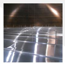
operation of the main structural elements. Additionally, Matrix Applied Technologies can provide a Hybrid IFR with the benefits of aluminum panels and stainless steel or anodized aluminum wetted parts.
